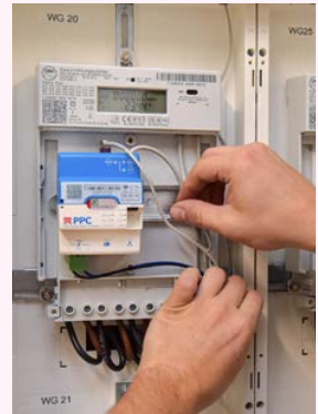
Smart-Meter-Installation.
